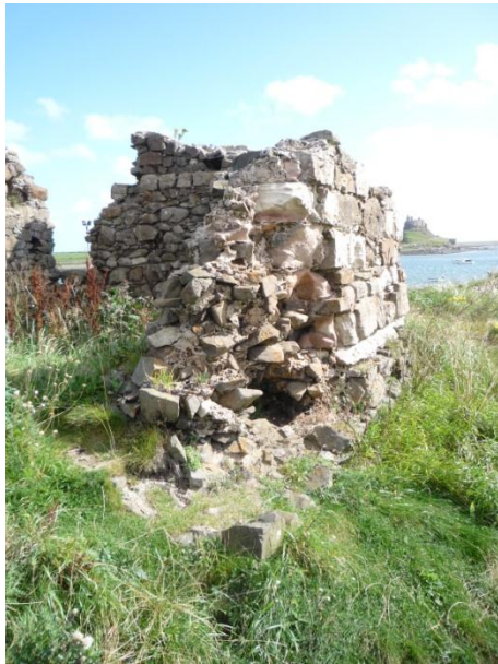
Illustration 35: Osborne's Fort showing deterioration of south east corner
